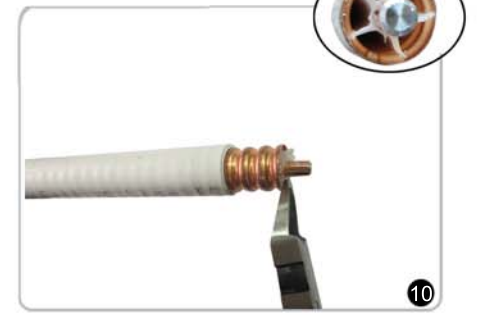
Remove the dielectric wings.
